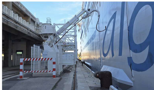
Ferries and ro-pax vessels – Various fixed CMS systems with 1 power cable – Marseille
