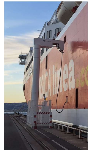
Ferries and ro-pax vessels – Various fixed CMS systems with 1 power cable – Marseille
