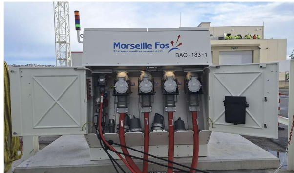
Cruises – Examples of PITs on the quays in Kiel and Marseille
