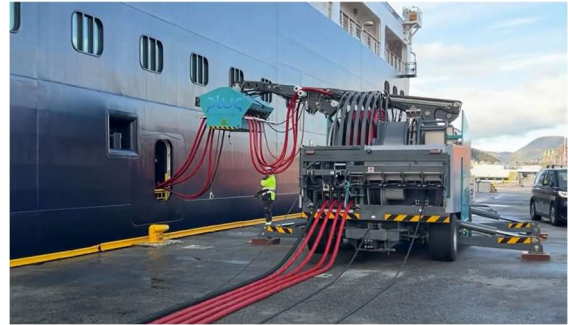
Cruises – Examples of mobile CMS with 7 cables, including 4 power cables – Southampton and Norway
