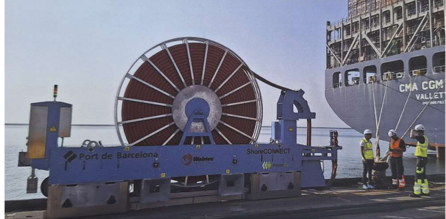
Sockets connected directly to the PIT Container ship with two cables connected on the quay
