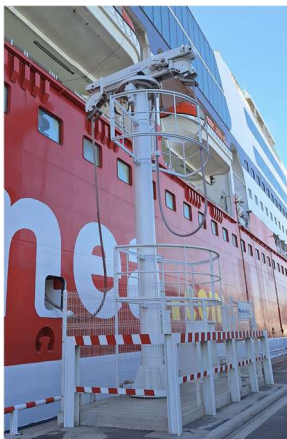
Ferries and ro-pax vessels – Various fixed CMS systems with 1 power cable – Marseille
